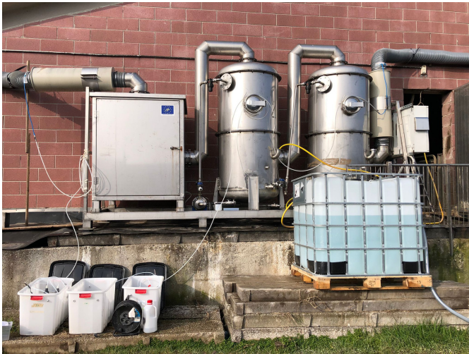
Fig. 9 Acid traps installation
